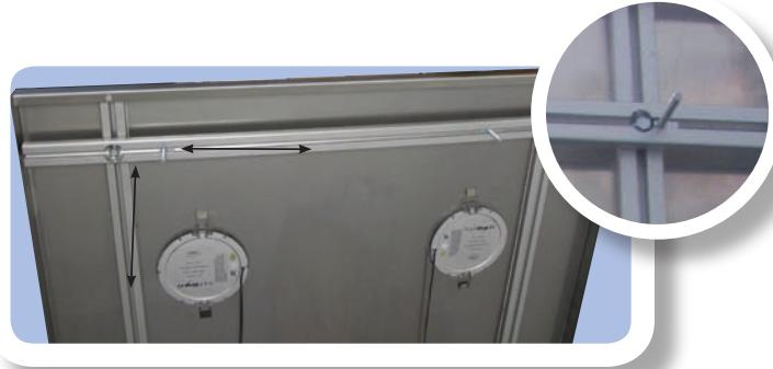
The pre-installed ceiling is fixed to the cabin roof with 4 threaded bolts.
