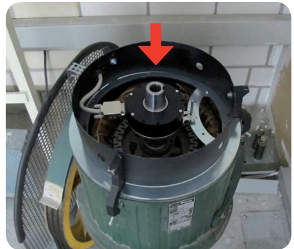
OTIS drive11VTR with encoder mounting
