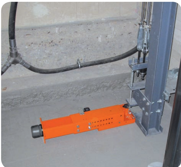
Examples: Fixation of the maintenance support at the piston support
