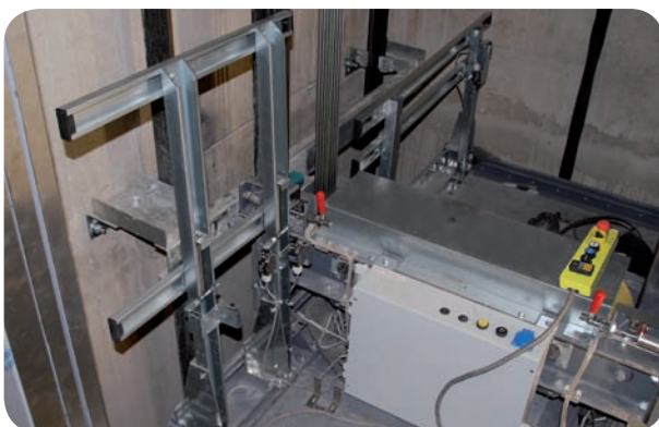
Mounting example: FOLDABLE and TELESCOPIC guard rail
