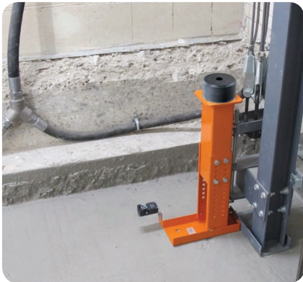
Examples: Fixation of the maintenance support at the piston support
