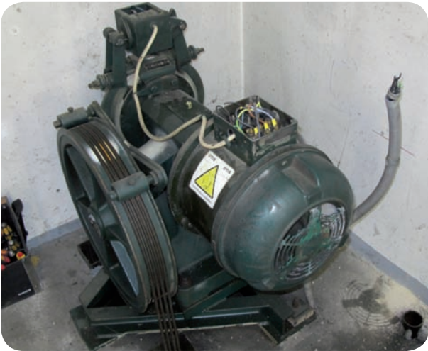
OTIS drive without encoder mounting
