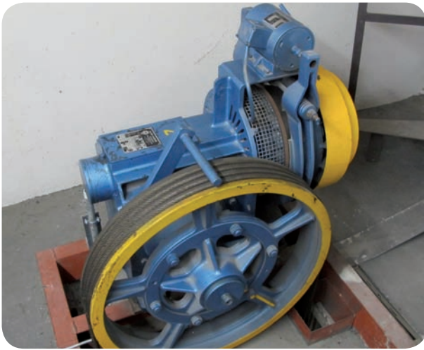
Example: KASPER drive KP120 without encoder mounting
