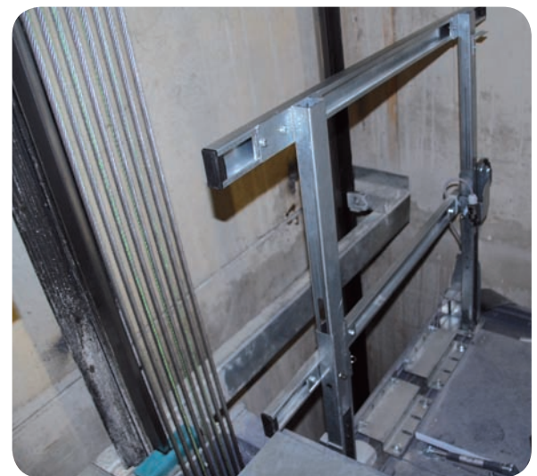
Mounting example: guard rail extended
