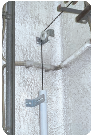
A Fixation diverter pulley on angle for roller fastening
